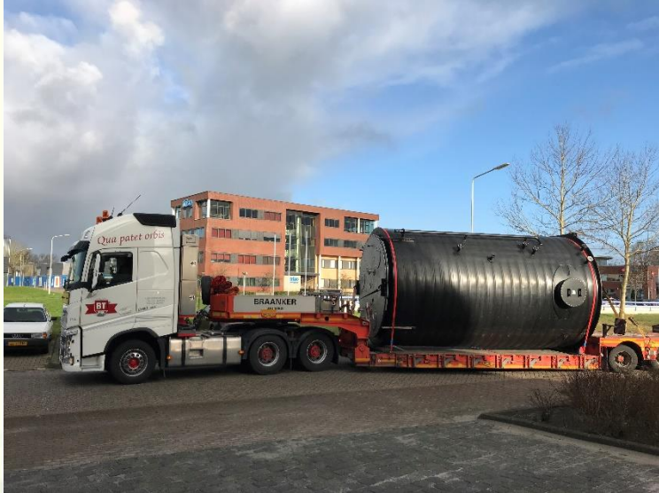
The Netherlands: Digester (office building Den Hage)
